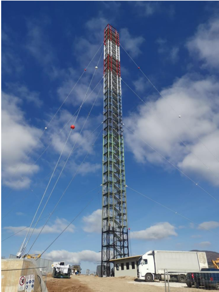
Figure 3. Picture of the Potenza ICOS atmosphere station under construction
