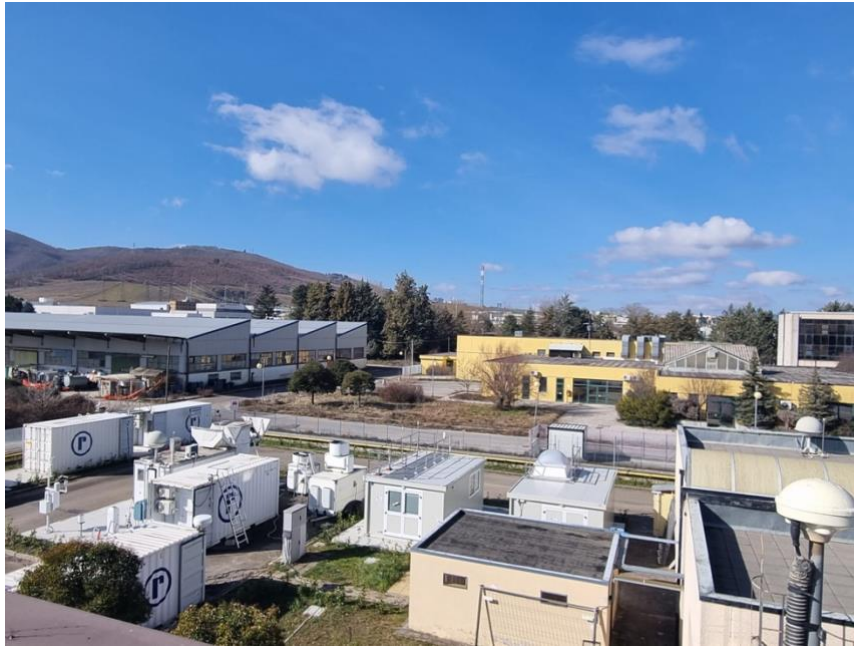
Figure 2. Picture of some of the measurement systems recently acquired and operational at CIAO
