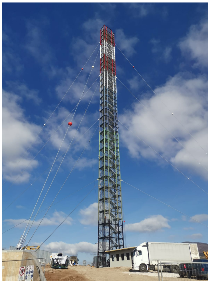
Figure 3: Picture of the Potenza ICOS atmosphere station during the construction phase.
