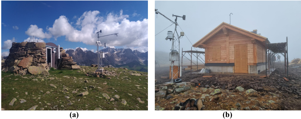
Figure 4 The high-altitude Col Margherita Observatory. (a) The old observatory, built inside an ISO 20' container, and the automatic weather station as of late summer 2023 (picture from CeTrA website). (b) The new building under construction as of Nov. 2024. The old weather station is still visible in front of the construction site.
