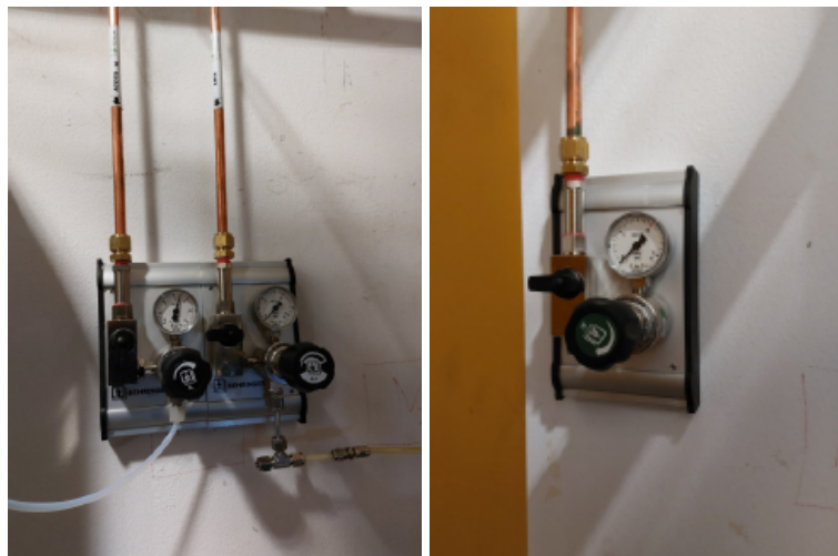
Figures 3 and 4: Access points inside the ChAMBRé room.
