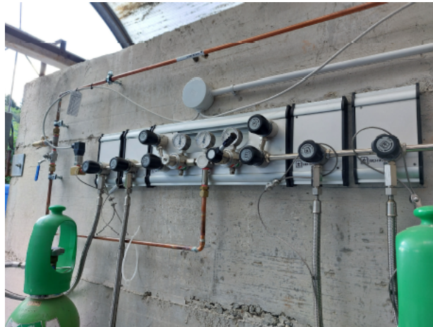
Figure 2: Automatic exchange decompression control unit for Air line.
