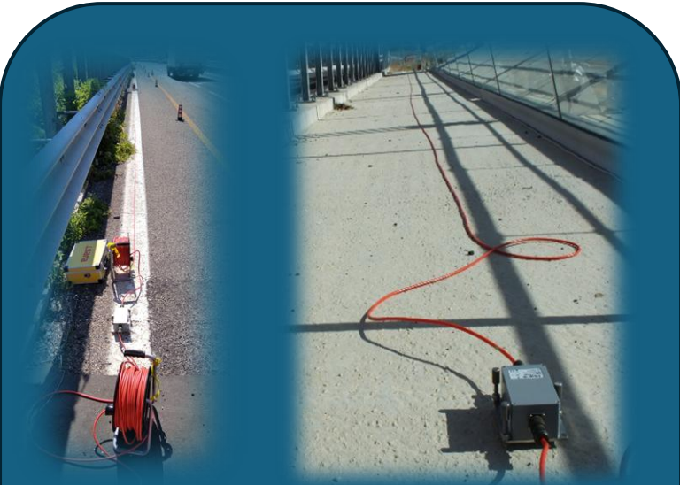
Strategic infrastructures characterization and monitoring
